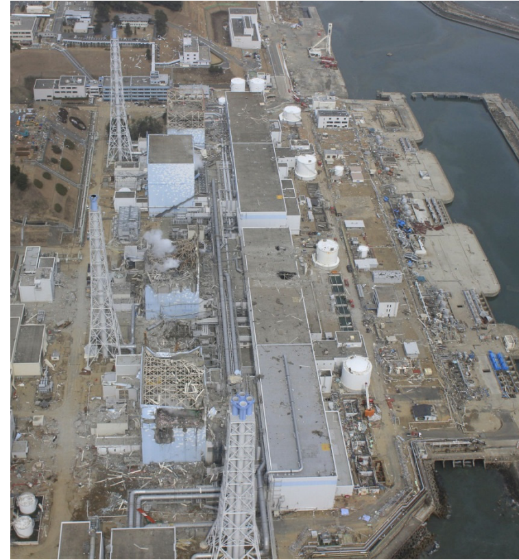
Fukushima Nuclear Power Plant after hydrogen explosion
