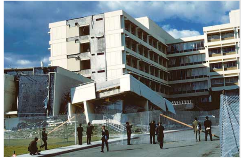
Damaged hospital in Sylmar during the San Fernando earthquake
