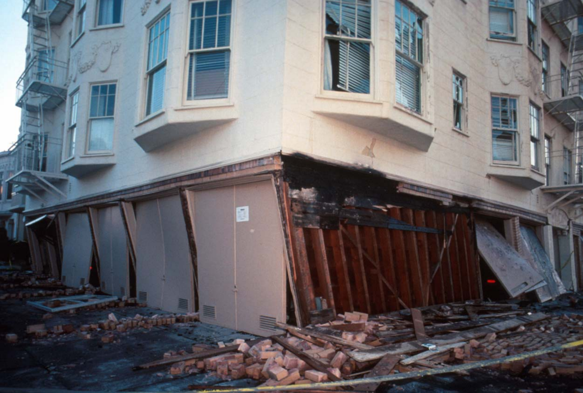
San Francisco, CA, Loma Prieta Earthquake 11/17/1989 Beach and Divisadero in the Marina District. U.S.G.S. by Nakata, J.K.
