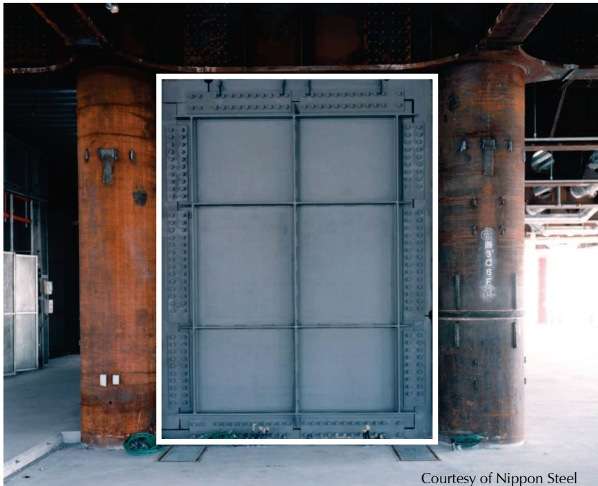
Figure 3-16 Illustration of a proposed component boundary for a steel plate shear wall in a seismic-force-resisting system (Sabelli, 2007).
