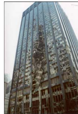
b. Deutsche Bank building [13]
