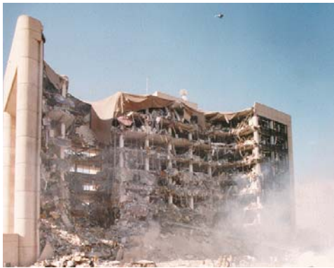
a. Murrah Federal Building
