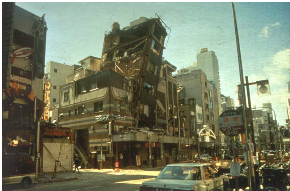
Figure 1: Buildings such as this office building in Kobe, Japan, are generally unstable and may collapse in an aftershock.
