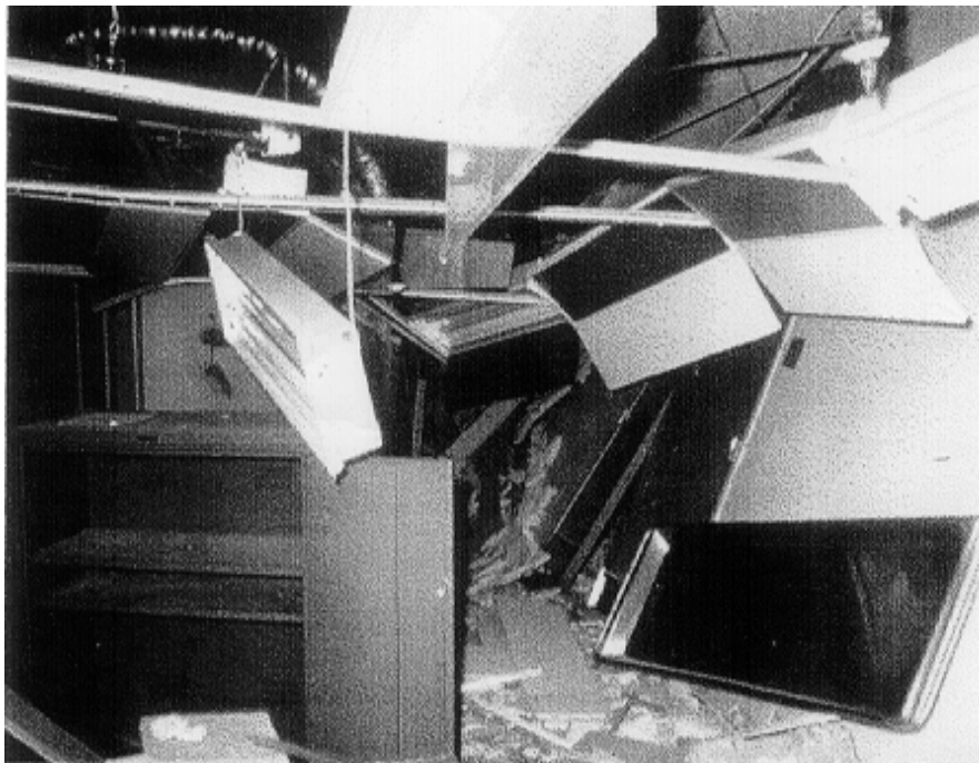
Figure 1. Earthquake Induced Partition Damage. Earthquake Engineering Research Institute photo.
