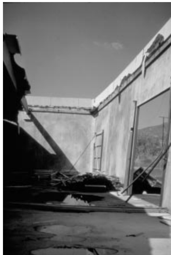
Figure 4. Concrete Tilt-Up Wall Building with Failure at the Wall-to-Roof Connection
