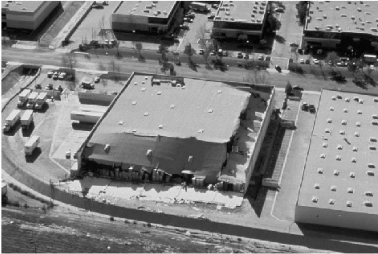
Figure 2. Failure of connection of wood diaphragm to concrete wall in Northridge earthquake
