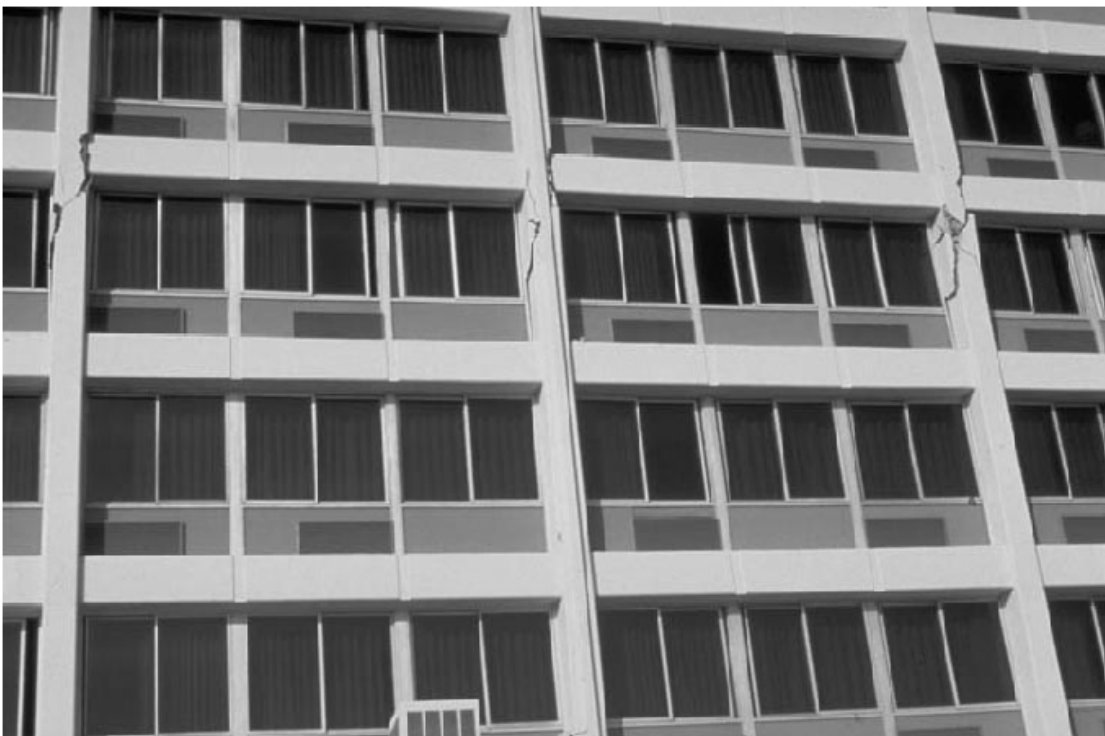
Figure 4. Beam-column joints damaged during 1994 Northridge earthquake.
