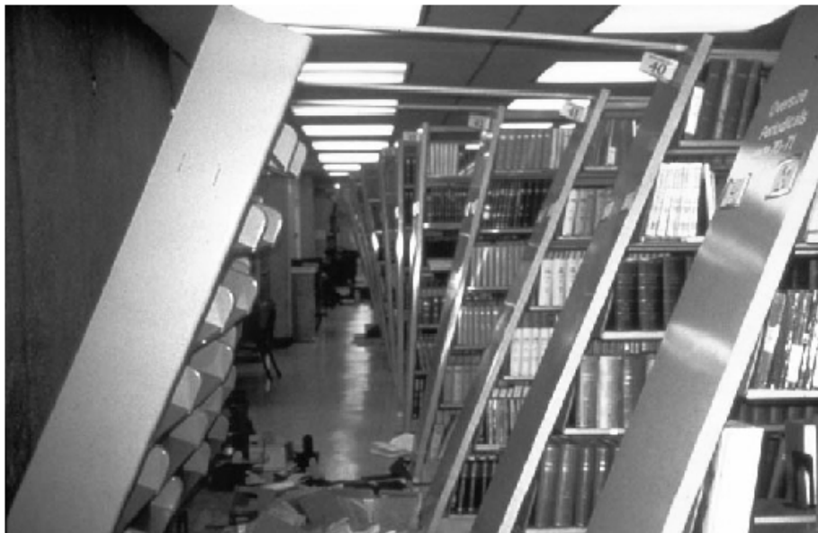
Figure 1. Earthquake-damaged book shelves (EERI photo).
